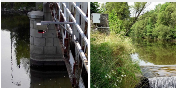
Flood warning system
